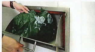
Inlets of refuse chutes
